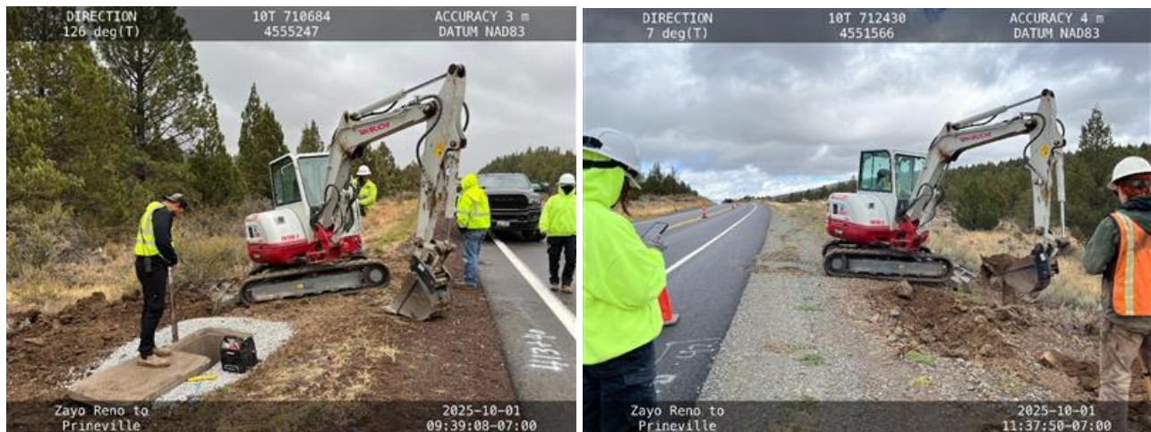
Figure 1. View of hand-hold operations in Northern Area (Lassen County).
